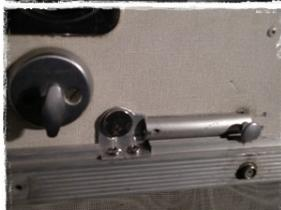
A single roller catch that holds the screen door closed is shown in the second picture. The flapper door, held by rollers, often rattles in the open or closed position.
