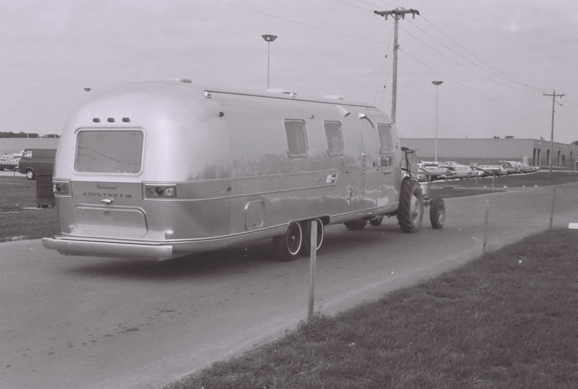
New Airstream plant in background nearing completion, not yet opened.
