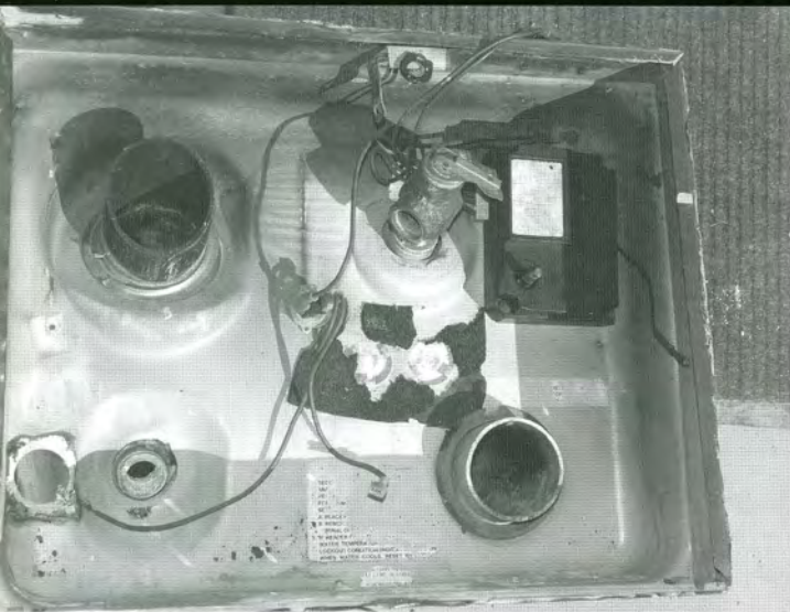
◀ Removing parts from the old heater
